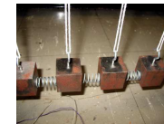
A few blocks in the middle section
